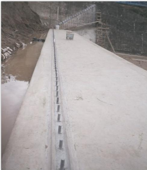
Figura 1.69. Placa embebida del dique inflable
