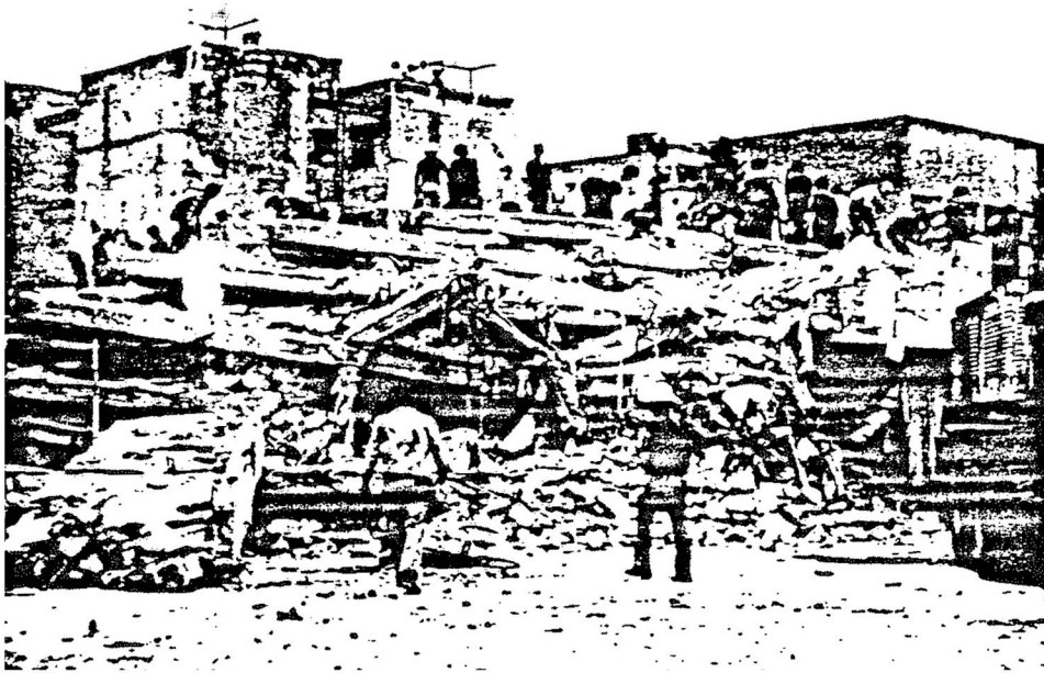
Colapso de edificio por inestabilidad lateral Collapse of building through lateral instability
