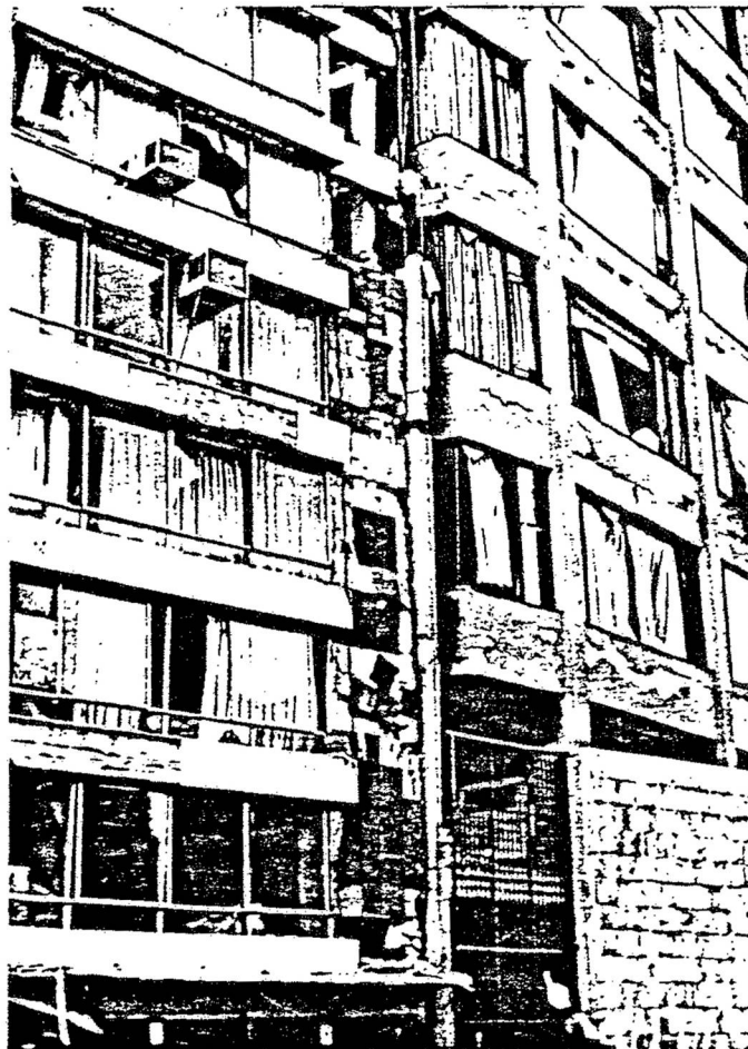
Daños por choques entre edificios adyacentes Damages caused by collision with adjacent buildings
